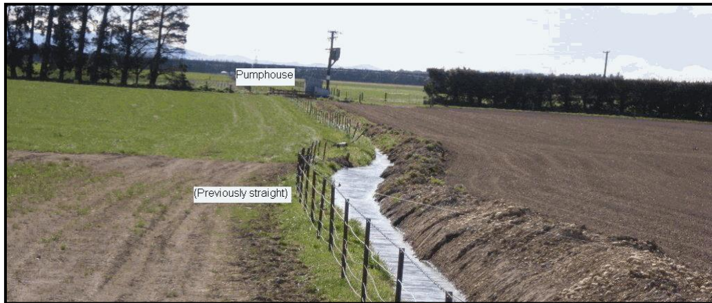
Figure 1 – Effects of fault rupture on previously straight fence and water race. (Photo - Survus Consultants)
